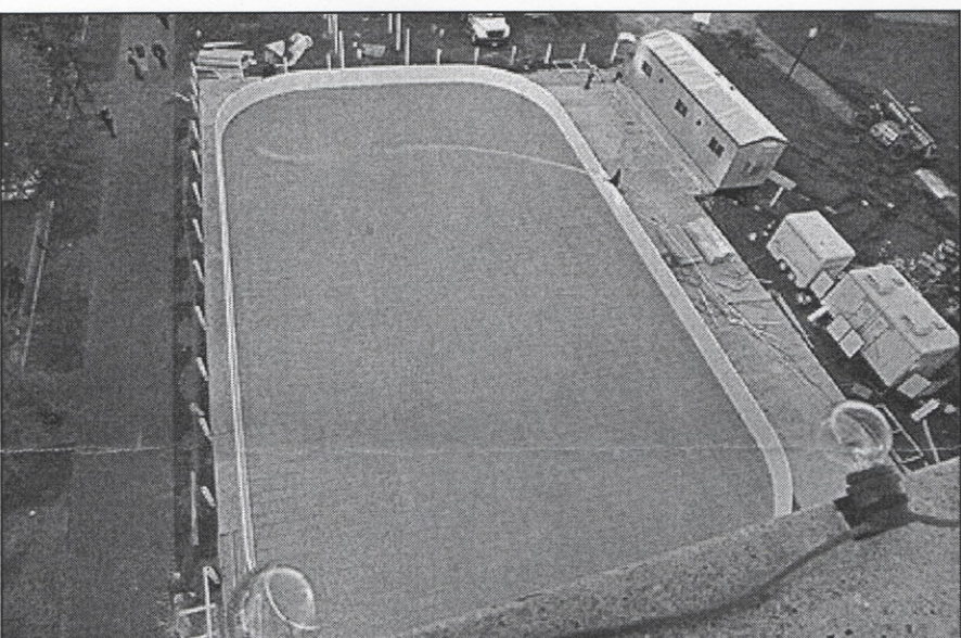
Water is frozen in layers and the chiller can keep the ice frozen as long as the temperature stays below 65 degrees, said Karen Winters, MacArthur Center spokeswoman. Up to 200 skaters will be able to occupy the rink. JOHN S. SHEALLY II/THE VIRGINIAN-PILOT
